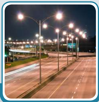
City Road Lighting
